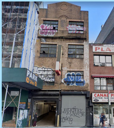
349 Canal Street/10 Wooster Street
